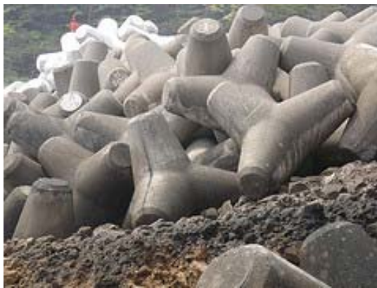
Tetrapods guard against Tsunami
